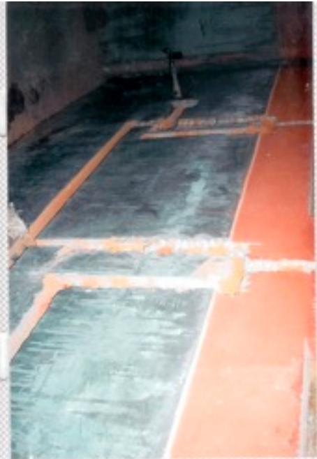
So the hot water is coming from left and cold water from right. They both join, and goes up on the tap.
